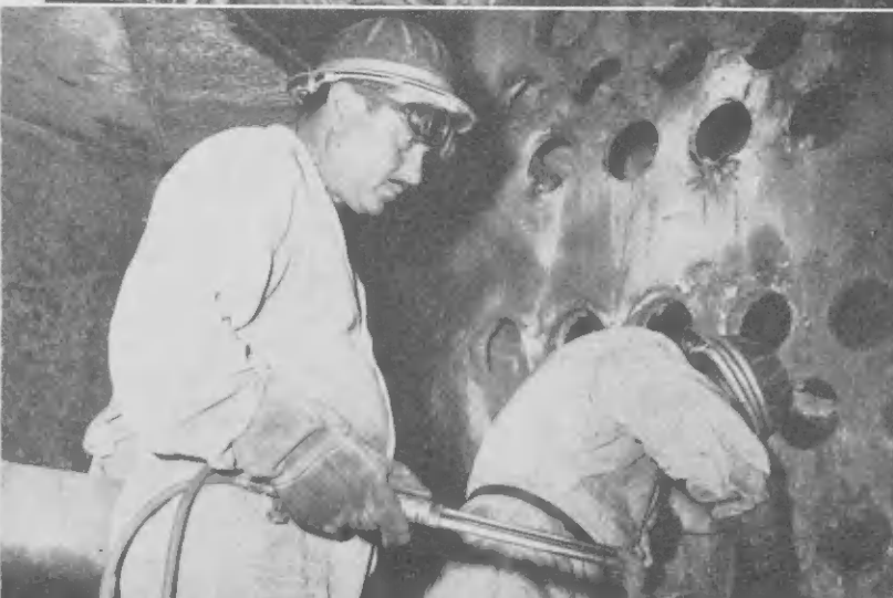
EVERYTHING GETS a careful going-over from valves to pumps. The convection section, left, its tubes pulled, is shown being cut up by workers. That face plate, right, will be lifted off by a derrick and the tube bundle inside pulled as part of the project to increase the visbreaker's efficiency of operating. About 320 men are involved.
